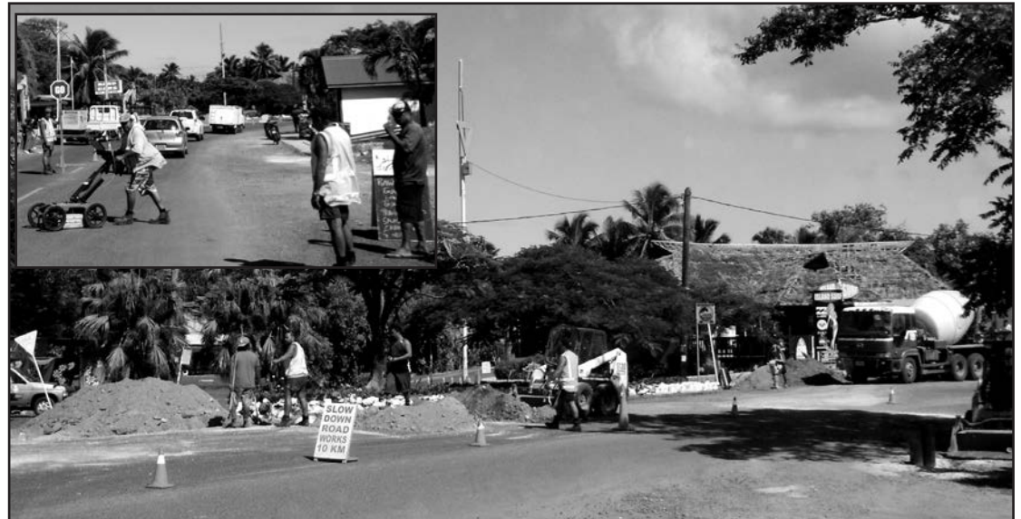
Bulk water-meter chamber being installed in front of Mamas Café Inset: Using the ground penetrating radar to locate service lines prior to trenching
